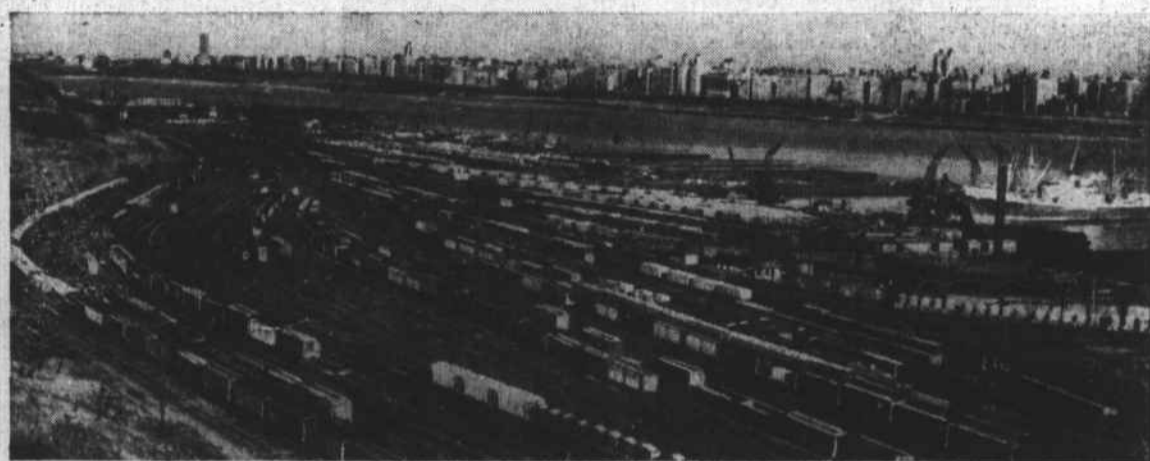
Central's huge freight terminal at Weehawken, N.J., opposite Manhattan, covers 140 acres, can hold some 5,000 cars.
