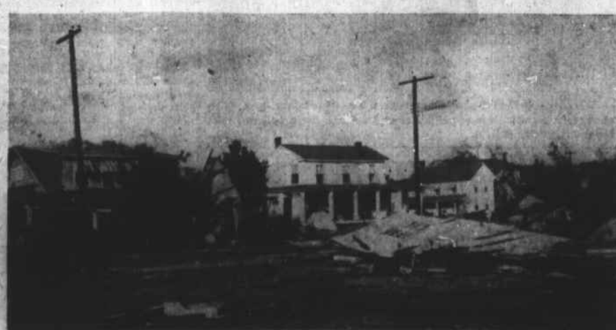
In the right foreground above is all that remains of the skating rink on Shepard Street in Morehead City. At the left a tin roof has crashed between two cedar trees, knocking down the porch of the brown-shingled house.
