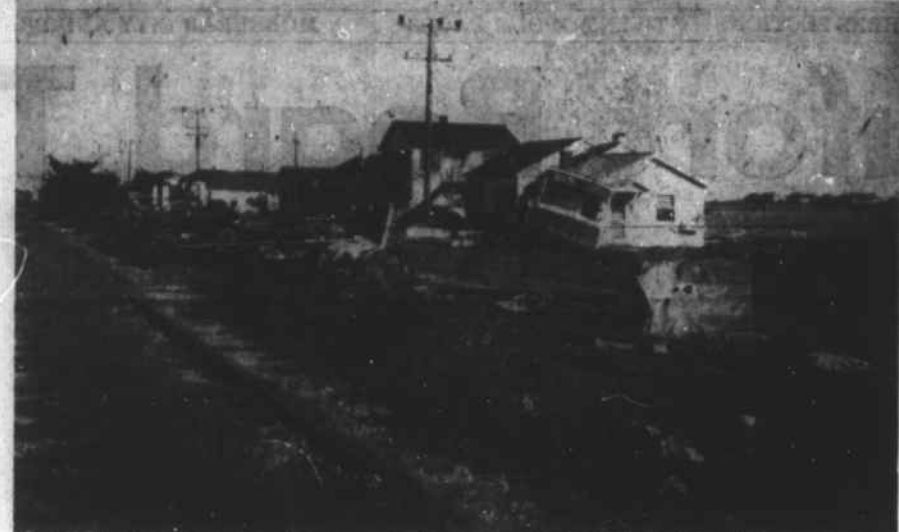
Looking southeast across the Beaufort-Morehead City causeway, the sightseer got an eyeful of the destruction property owners withstood there.
