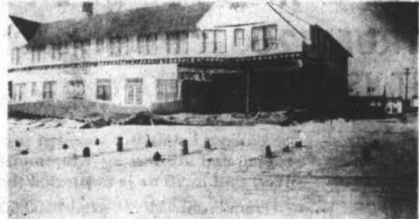
The Atlantic Beach Hotel lost its front porch, boardwalk and dining room walls in the storm.
