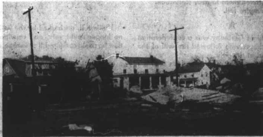
In the right foreground above is all that remains of the skating rink on Shepard Street in Morehead City. At the left a tin roof has crashed between the two cedar trees, knocking down the porch of the brown-shingled house. (More pictures appear on page 6).
