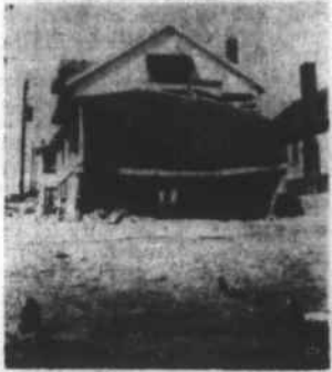
Typical of many of the ocean front cottages is this one with a collapsed front. Many others were more severely damaged.
