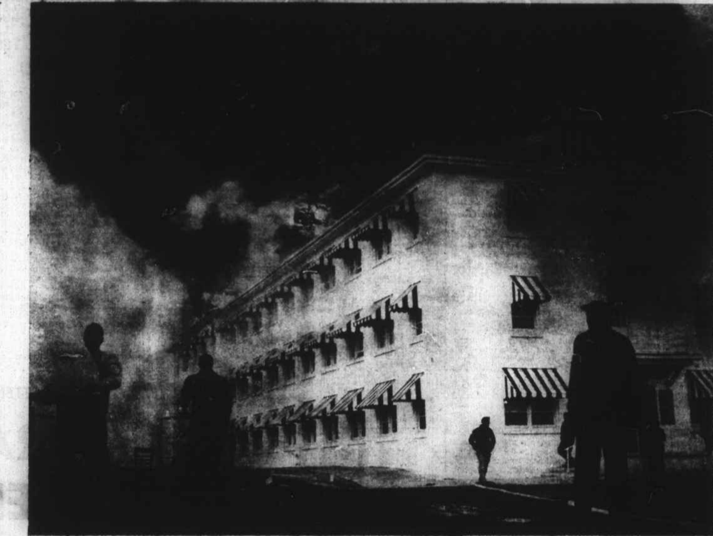
Smoke billowed from the Ocean King Hotel at 7 o'clock yesterday morning. Flames ate their way from frame buildings west of the hotel and into the concrete block structure. At left is James Jones, Morehead City bellboy, who noticed the wooden buildings ablaze and gave the alarm. This picture shows the back of the hotel on the landside. The hose line in the foreground was run to Bogue Sound to get water. The fire is believed to have started in a building to the right of this picture. Photo by Clifton Guthrie
