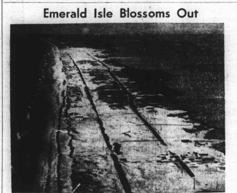
Among the busier Carteret beach spots these days is Emerald Isle, located west of Salter Path. Four new homes have been built, 10 are in process of completion and construction of 20 more is scheduled to start before July 1.
