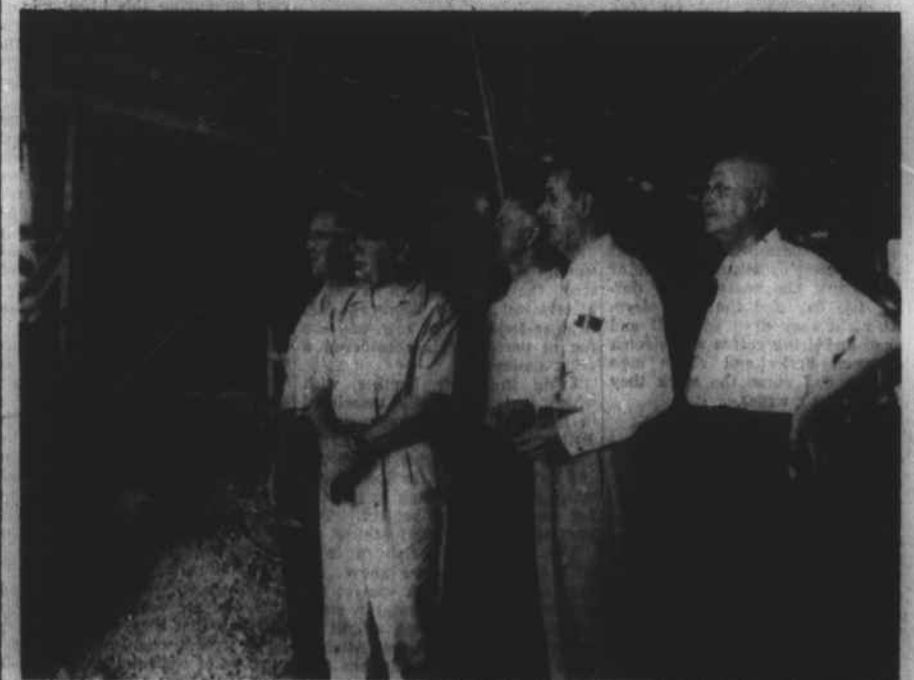
Gov. Luther H. Hodges (the man wearing the cap) was a recent visitor to the huge trawler shed of the Morehead City Shipbuilding Corp. It is under this shed that the construction begins. Six of the new famous fishing craft can be constructed under this shed at the same time. R. C. Kirchofer, president of the corporation, second from right, is explaining the operation to Governor Hodges.
