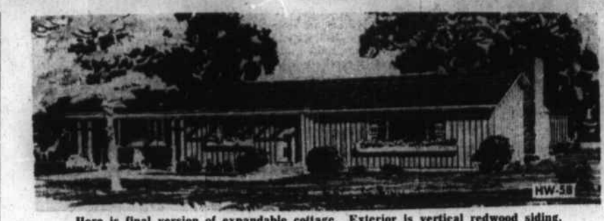
Here is final version of expandable cottage. Exterior is vertical redwood siding.
