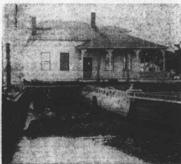
Getting a house from dry land, across a sea wall to a barge, is a neat trick if you can do it. Here it's being done!
