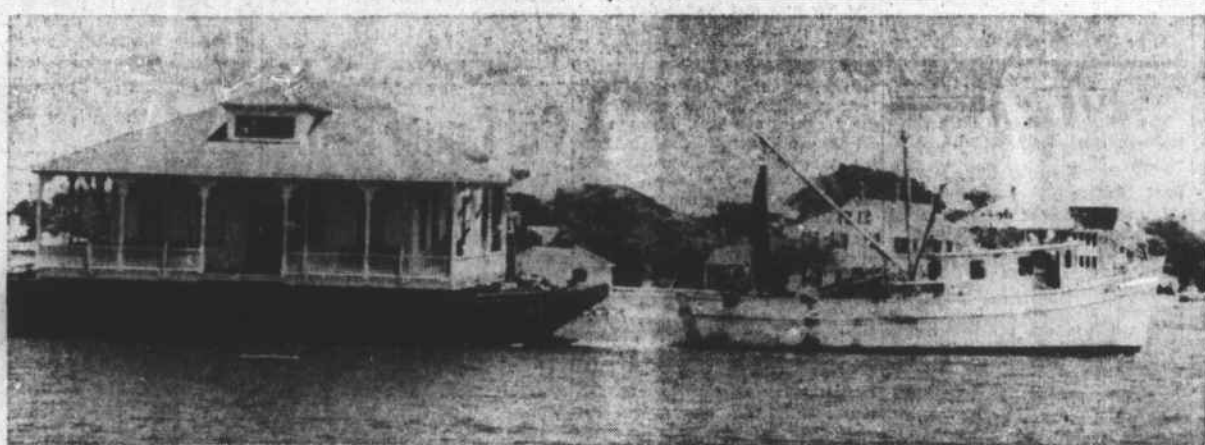
Here goes the house, south on Gallants Channel, towed by the shrimper, Allie A. In the background is the west end of Front Street, Beaufort.
