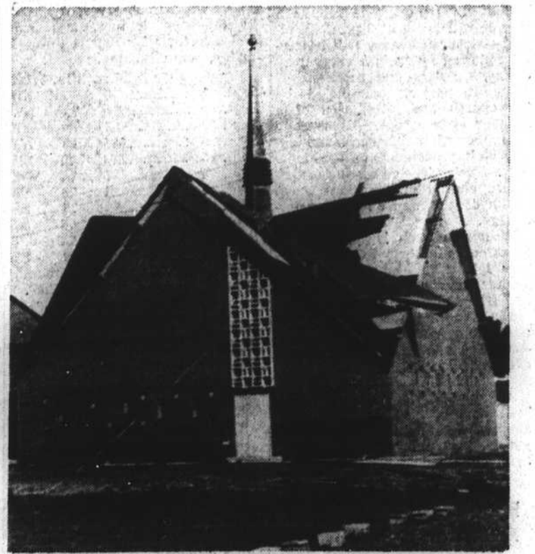
Donna's winds rolled together sections of the copper roof on the new chapel of the Church of Jesus Christ of Latter-Day Saints on Harkers Island. Dedication of the chapel, scheduled for Sunday, has been postponed.
