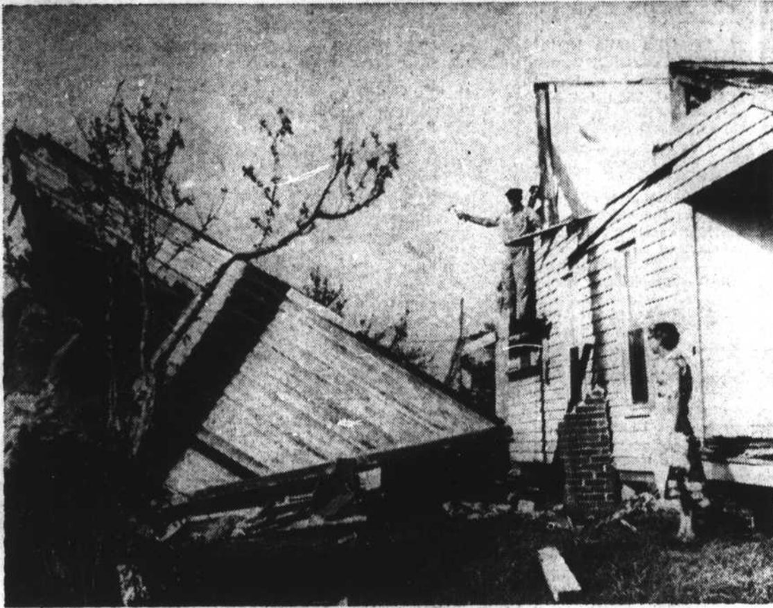
The Oliver Chadwick home, Gloucester, lost its roof in a twister that arrived about five hours before the height of the storm. Mr. Chadwick points with a hammer in the direction of the route taken by another roof which was on the side of the house opposite the side pictured. Mrs. Chadwick is at the right.
