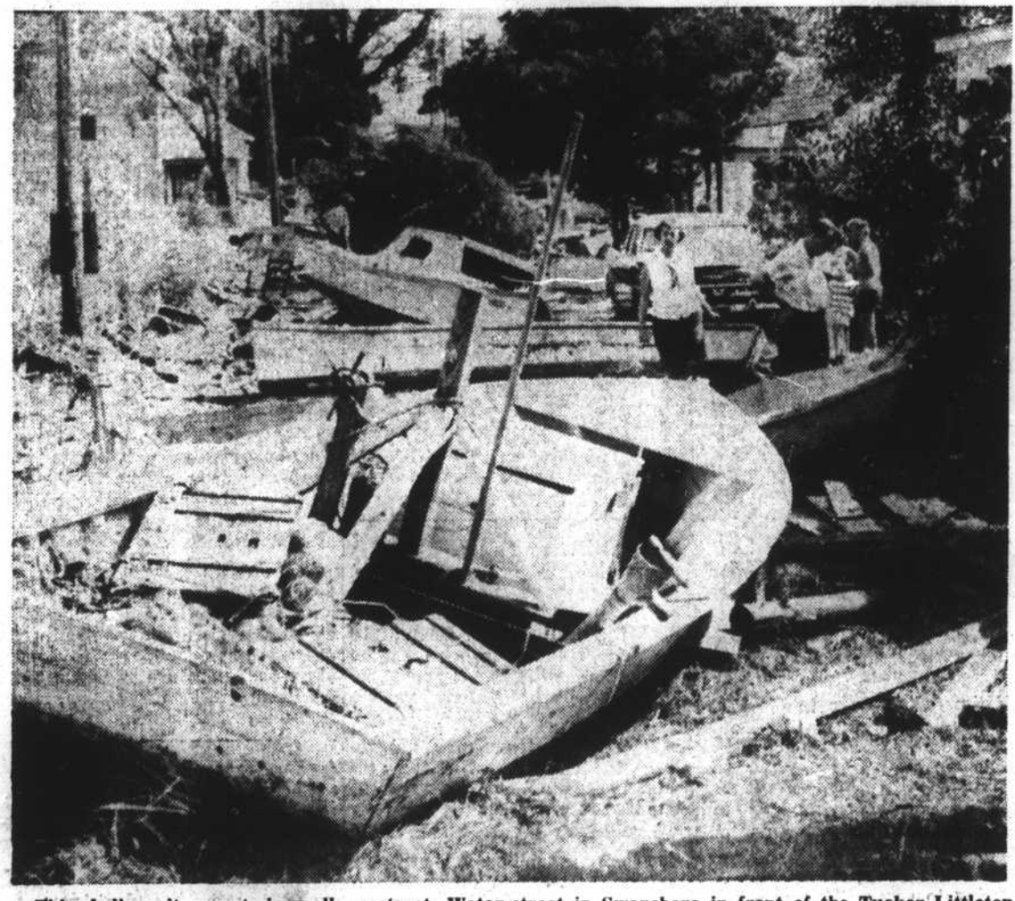
This, believe it or not, is really a street, Water street in Swansboro in front of the Tucker Littleton house, looking east. (Photo by S. F. Milsted.)
