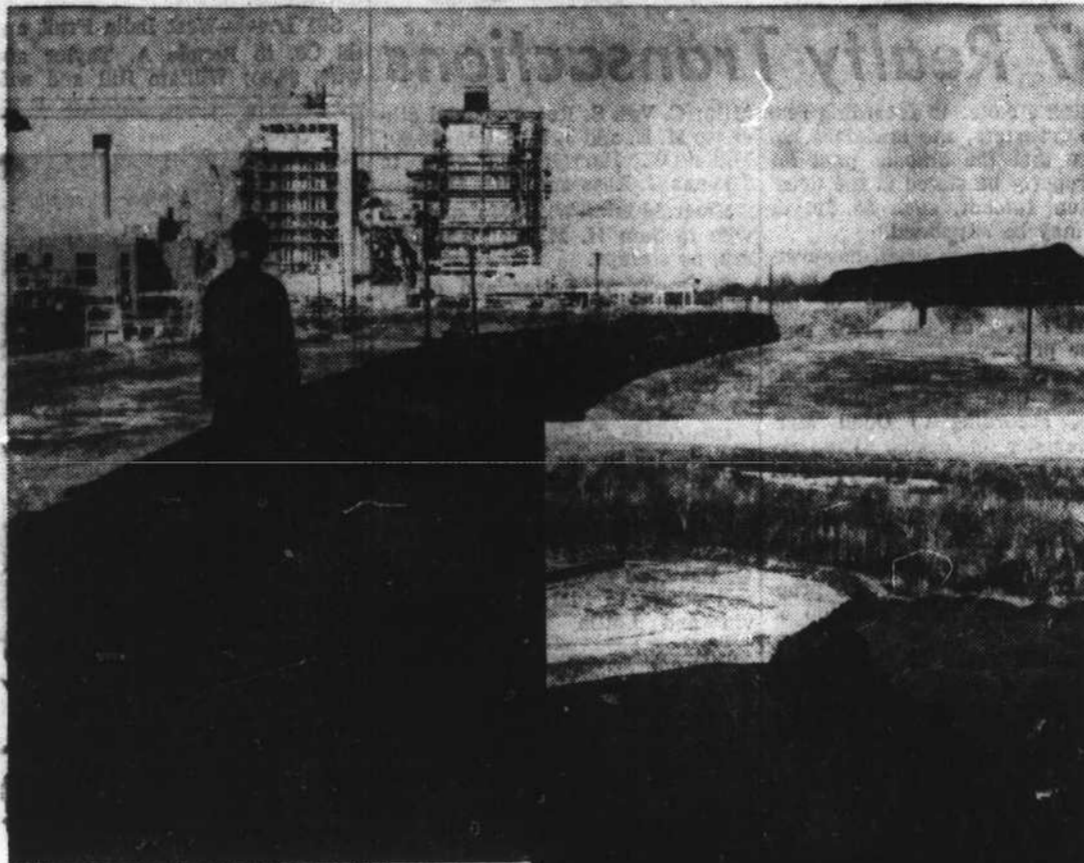
Fifteen rail cars of coal head into Carolina Power and Light company's Cape Fear steam-electric generating plant near Moncure, N. C. This shipment, about 1,350 tons, will supply the plant for eight hours. Inset, a bulldozer and coal cars are dwarfed by the gigantic 115,000-ton coal reserve at the Cape Fear plant. Here coal is converted into electricity — "coal by wire" — to serve CP&L customers in the two Carolinas.
