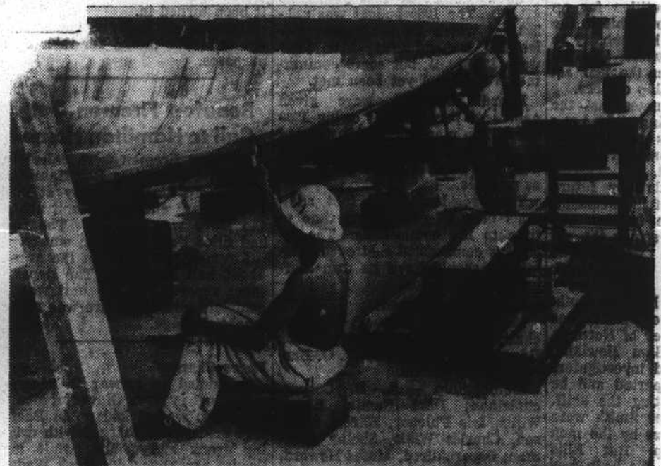
Skilled Cuban laborers work on Navy ships at repair base.
