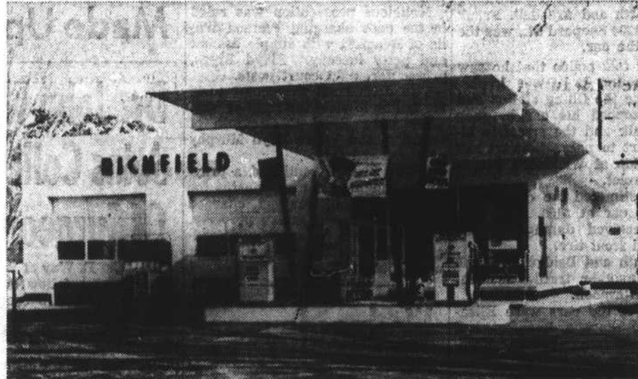
Bill's Richfield Service Center
