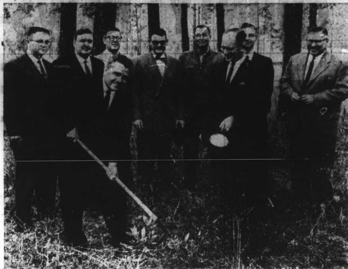
Ground was broken Wednesday at a Forest Hills site for a Paragon home to be erected by the Med-law Corp. of Morehead City. Doing the digging is Daniel Greenhauff, president of Paragon, from Mine-ola, Long Island. At his left is mayor George Dill, Morehead City. Others taking part in the ceremony, left to right, are Garland Scruggs, Luther Hamilton Jr., Rufus Butner, Dr. Silas Thorne, Cleo Merrill Herbert Phillips and H. Earle Mobley.
