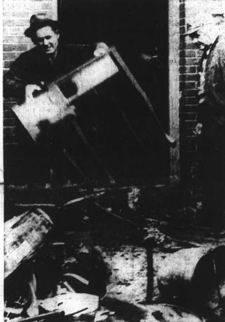
At the rear of the store, fire chief Lindsey Guthrie, right, directs removal of furniture so that firemen can work more efficiently. Mart Bell, fireman, is carrying out the table. Fire is believed to have started around a light fixture.
