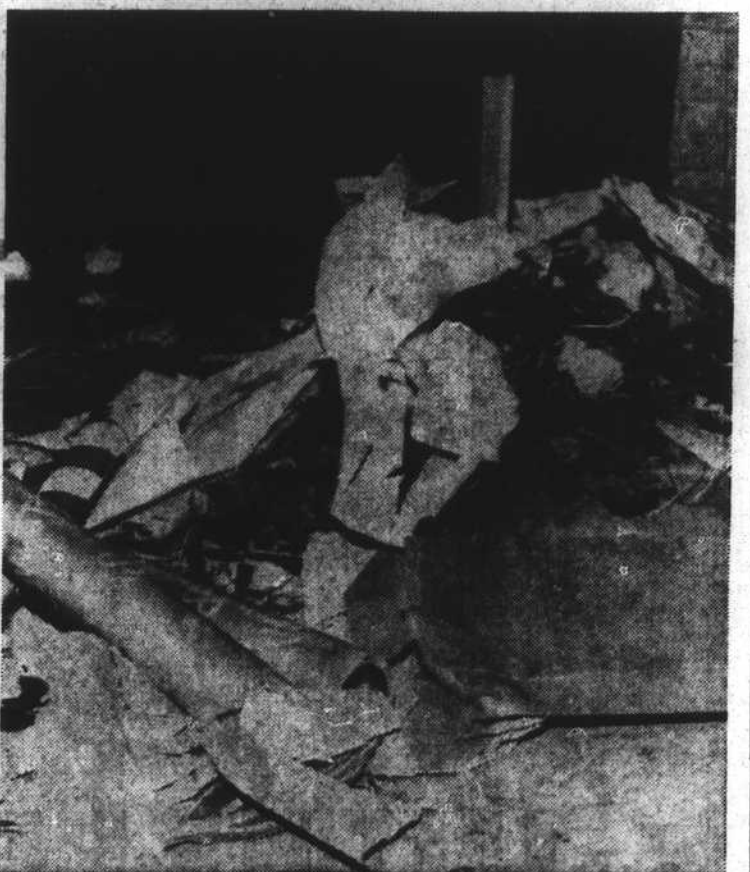
This is a heap of trash backstage at the Morehead City recreation building . . . a good place for fire to start. The trash is the remainder of a recent school affair at the building. Students like to decorate for a dance, but don't like to clean up afterwards. Tomorrow is the last day of a current county-wide clean-up campaign.
