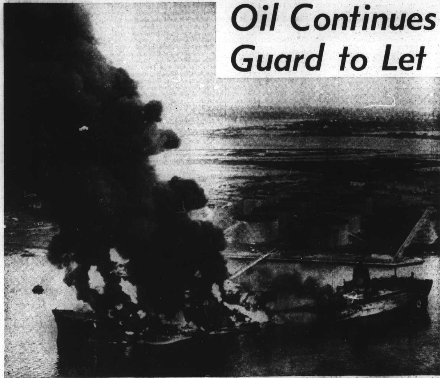
The Military Sea Transport Service tanker, USNS Potomac, still blazes brightly almost 14 hours after it exploded and started burning at 6:45 Tuesday night. The tanker was loaded with four-and-a-half million gallons of aviation fuel. At the time of the fire, the fuel was being pumped from the ship into fuel storage tanks, also containing aviation fuel, located about 550 feet from the ship. While the ship continues to burn, firemen keep a spray of water going on the two forward storage tanks to keep them cool. In the background is Beaufort.
