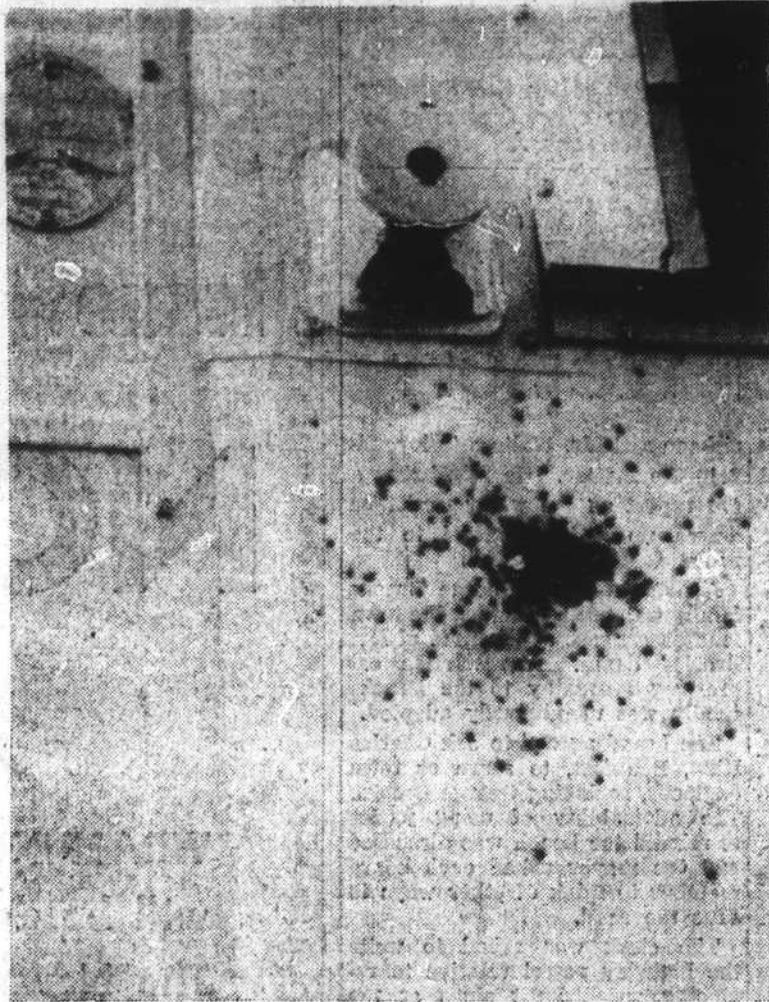
This is the door of the Rodney Gaskill trailer, where the first shotgun blast entered.
