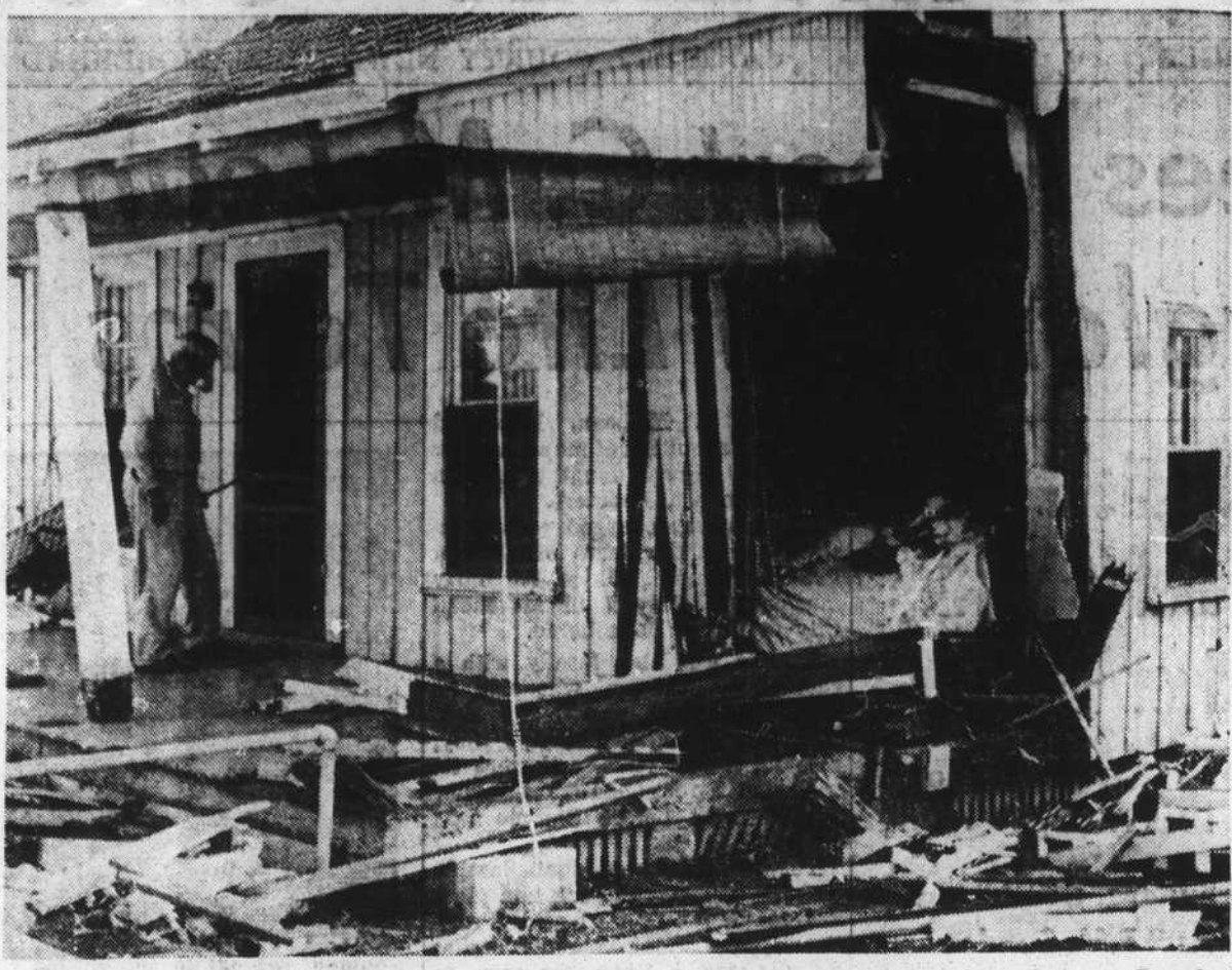
This is one of the two homes badly damaged when a runaway car plowed into them at Beaufort Friday. The car took off both the front porch and a corner of a front room. The home is that of Henry Styron, 506 Broad St. Mr. Styron is on the front porch.
