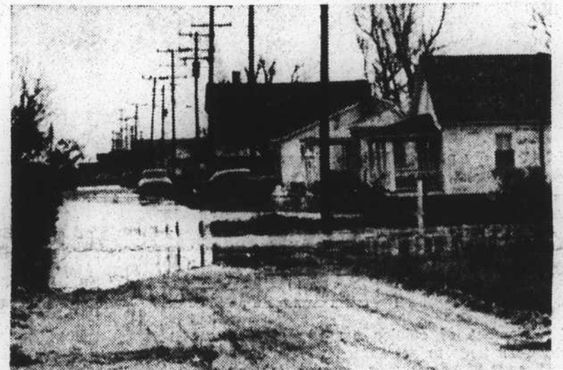
Areas exposed to the north were flooded. This is a view on Bay street and 9th, Morehead City. John Dozier, 809 Bay, when asked if he had any damage from the storm, said, "Damage! Why the water's so high in my yard the hogfish is eatin' the collards."
