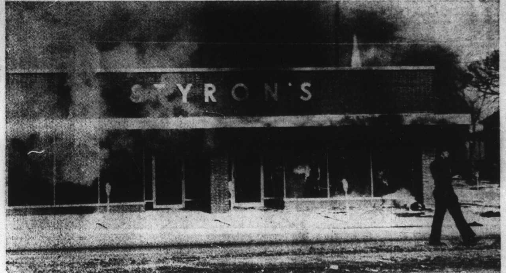
Flames lick at the interior of Styron's Department Store Wednesday at the beginning of a fire that gutted the building. This picture, taken just after the blaze was discovered and before firemen arrived, shows a smoking show window mannequin at the right hand corner of the building. The dummy and some of the clothing in the store window was spewed out on the sidewalk as heat and pressure from the fire blew out store window glass.
