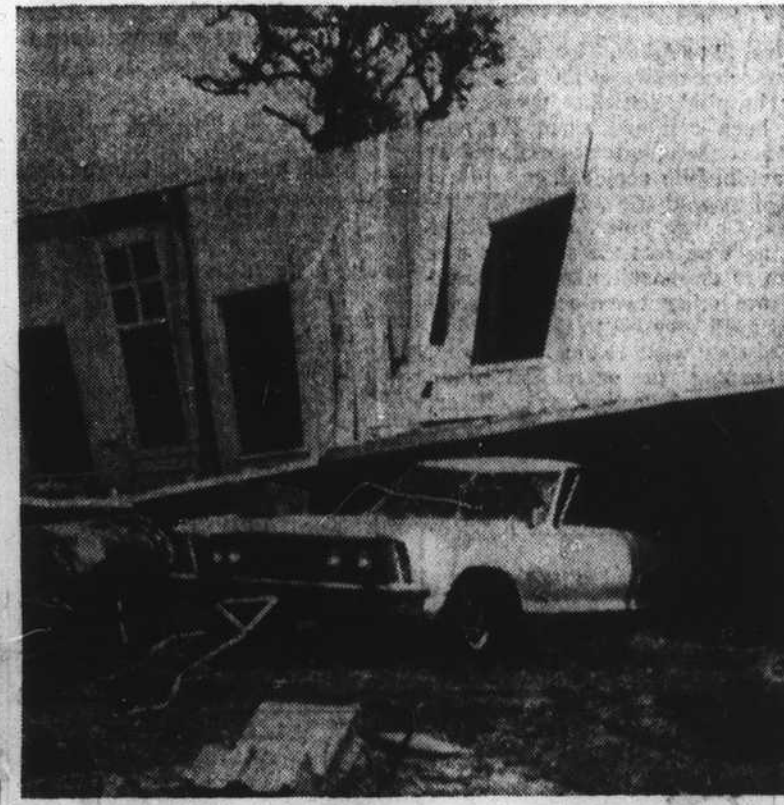
The 1963 Buick Riviera belonging to Mr. and Mrs. Jimmy Chappell was crushed by the weight of the frame cottage. The cottage roof is resting on the automobile, with the floor pointing skyward.
