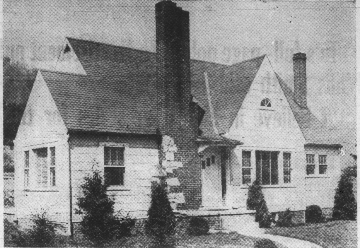
Home of Mr. and Mrs. Stanley Riddle in West Burnsville. It is of asbestos siding and of story and half construction, built in 1946
