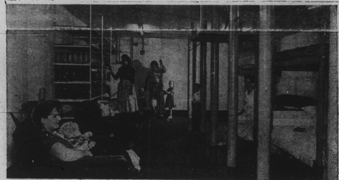
THE ULTIMATE in family shelters is represented by this large and luxurious unit built by steel contractor Earl W. Reichert of Battle Creek, Michigan. The $10,000 structure has a 98-foot well, private electric generating plant, electric and hand-operated blowers for the filtered air system. Its steel reinforcement prepares it for use as a blast as well as fallout shelter. However, a small family fallout shelter may be built for a fraction of what this shelter cost. (Battle Creek Enquirer and News Photo)
