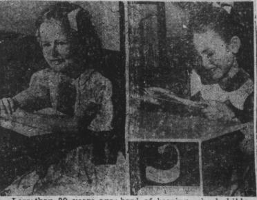
Less than 20 years ago, hard of hearing school children wore heavy, bulky vacuum tube hearing aids (left) with separate battery case at hip. Today, new miniature ear-level aid (see inset) designed by Zenith Radio Corporation fits behind ear of six year-old child, contains small mercurybattery, and weighs one-third of an ounce!
