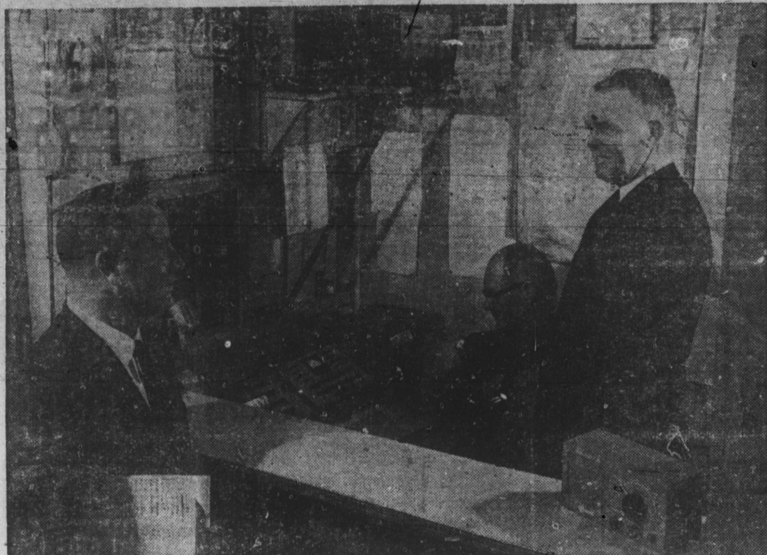
COMMUNICATIONS CENTER at Wadesboro, N. C., combines a round-the-clock civil defense nerve center with a unified radio service for local police, fire and sheriff's departments. Used for this dual purpose, the equipment is kept in top-notch condition at all times to meet emergencies. At the radio is Waldo J. Stroud, one of three operators hired by the local CD unit under a program in which Federal and local governments share the costs of new civil defense employees. Raymond H. Northcutt (right), Wadesboro-Anson County CD director, explains his radio setup to Herman J. Sisk, Area E director for the North Carolina Civil Defense Agency and one of five area directors hired under the same cost-sharing law to help build up CD at the local level. (OCDM Photo)
