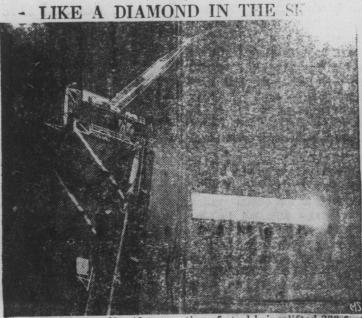
Sun glistens off a 40-ton section of steel being lifted 200 feet into air to form part of nation's newest monum construction in St. Louis, fabulous Gateway Arch will rise 630 -75 feet higher than Washington Monument. When completed next year, its gleaming surface will be visible for 30 miles. Arch was designed in stainless and other types of modern steels by late Eero Saarinen as enduring tribute to pioneers who pushed westward in last two centuries.
