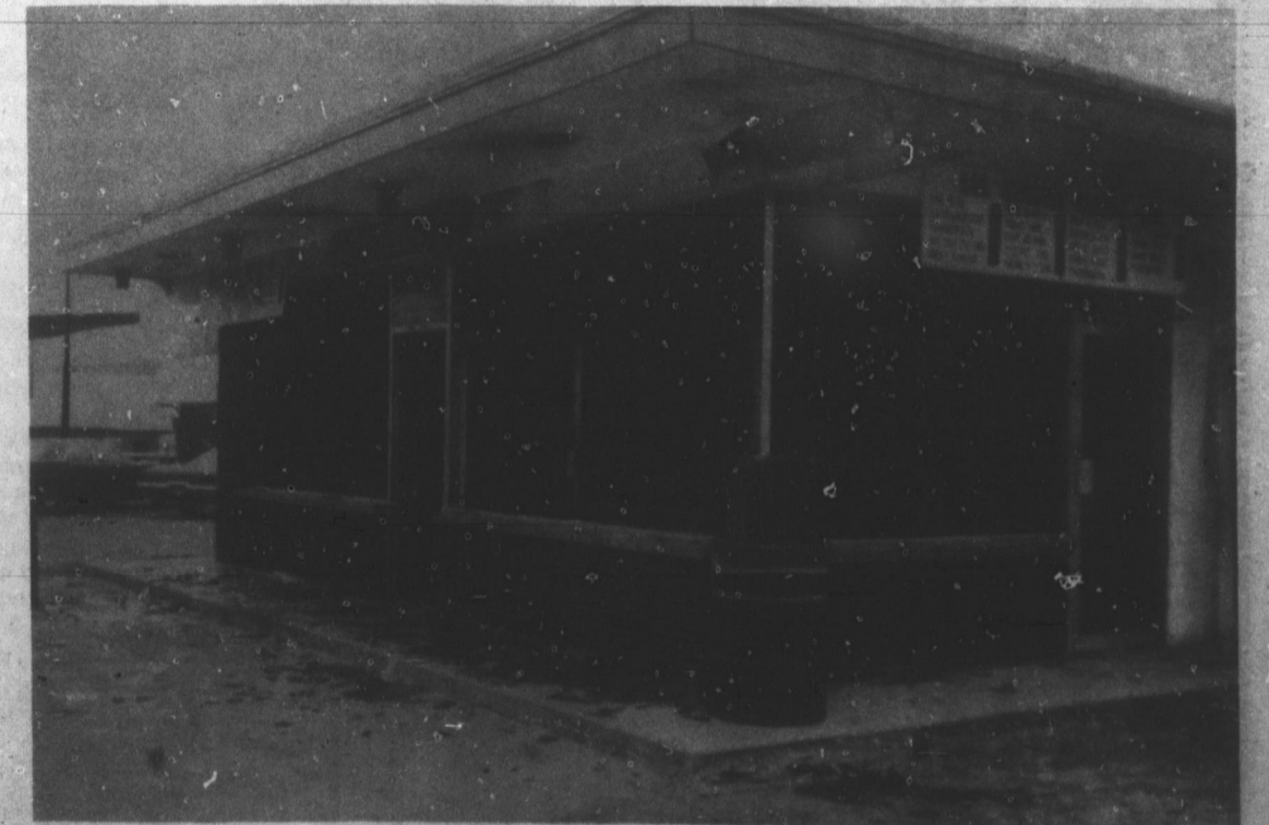
Li'l Smokeys Damaged By Blaze
