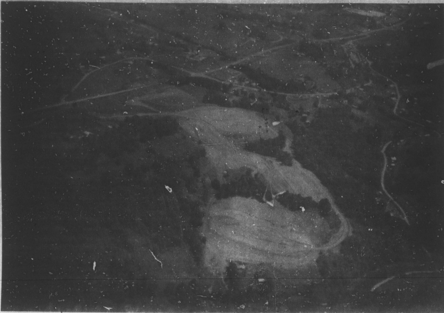
Aerial View Shows Excavation At Site Of New Mountain Heritage High School
