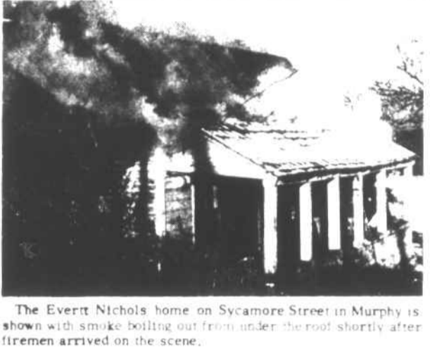
The Everett Nichols home on Sycamore Street in Murphy is shown with smoke boiling out from under the roof shortly after firemen arrived on the scene.
