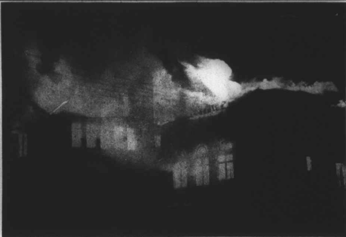
FLAMES completely destroyed the Andrews High School building early Tuesday morning. This picture was taken at the height of the fire around 4:40 a.m. As the Scout photographer topped the hill in front of C. H. Townson's house on U. S. 19,
