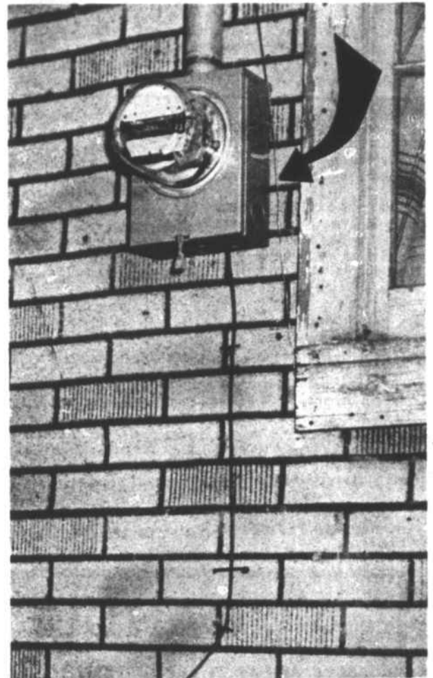
ARROW SHOWS piece of ordinary clothesline wire by-passing the electrical meter at the Isaac Thompson home. For this small piece of wire that served no useful purpose, the con artist trio received $91.00.
