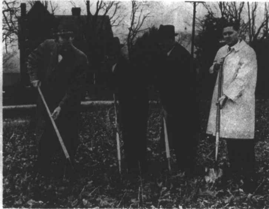
GROUND BREAKING- Those participating in the actual ground breaking for the new Federal and Post Office Building in Andrews were (L-R) Percy B. Ferebee, Mayor of Andrews, James O. Trogdon, General contractor, W. T. Martin, Postal Service Officer, and A. D. Johnson, Architect. Photo by Scout Studio
