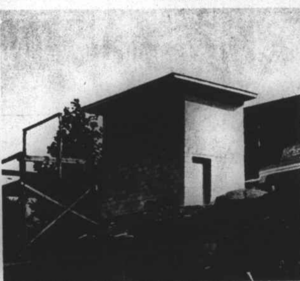
THE NEW PRESS BOX AND RESTROOMS at the Murphy High School Football Field is almost completed. The press box will definitely be in operation for Friday night's home game. Construction problems may delay opening the restrooms but Quarterback Club officials stated that if at all possible the entire facility will be open Friday night.
