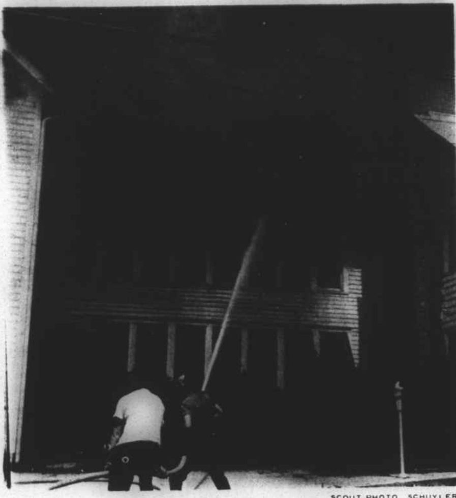
FIREMEN PLAY A STREAM of water on Murphy's Historic Henry House Sunday afternoon. The smoke rising in the background was visible for miles around the town.
