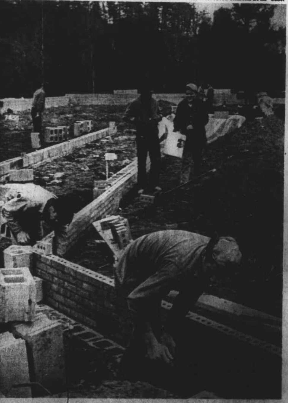
New Baptist Church Construction
