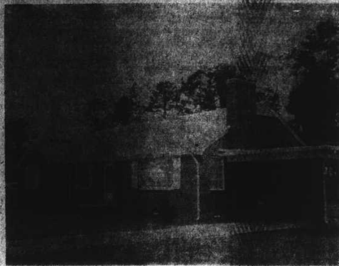
This is the new Methodist Parsonage at Maysville which was recently completed and is now the home of The Reverend and Mrs. Robert F. Moore. Built at a cost of something more than $16,000 the new home is modern throughout and is located in the Southern end of Maysville, one block west of the Main Street.
