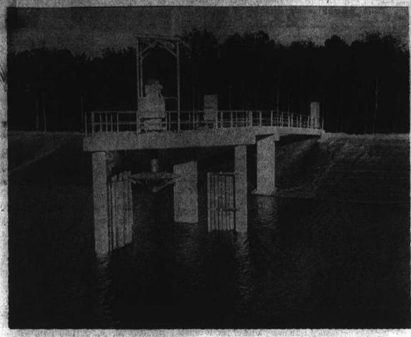
This picture shows one corner of the 6million-gallon aeration chamber of the Kinston Sewage Treatment facility which is now nearing completion and includes a view of one of the six aeration propellers in the chamber. This is likely to be the last time
