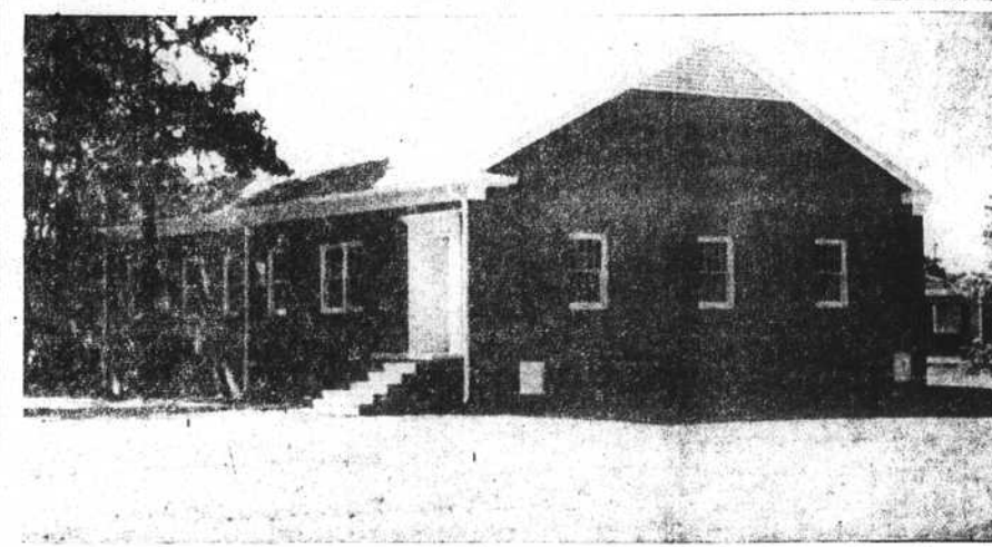
The above picture of the new Sunday school building just completed by the Page Memorial Methodist Church and located between Highway 1 and Poplar street. This new addition was added on to the Sunday school building across from the Methodist Church and is 70 feet long and 41 feet wide. The addition, constructed with brick and slag blocks, has six class rooms, three toilets, a utility room and a hall. The old building to which the new addition was attached has beautiful and conveniently arranged and can be entered from a side back door as shown in the above picture or from the front facing Poplar street. Members of the building committee were: F. D. Shamburger, chairman, Mrs. Forrest Lockey, Mrs. R. S. Gwyn, Mrs. Mack Wallace, Morris Greer, Leo Arty, D. P. Troutman, Ralph Chapman and E. B. Satterwhite.—Citizen photo.
