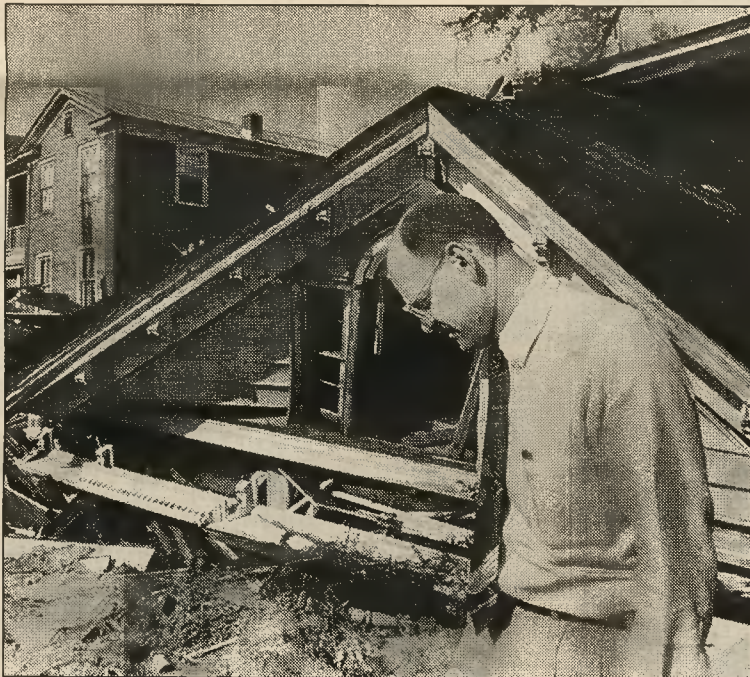
Charles Chase stands by his collapsed home in Charleston, SC.
