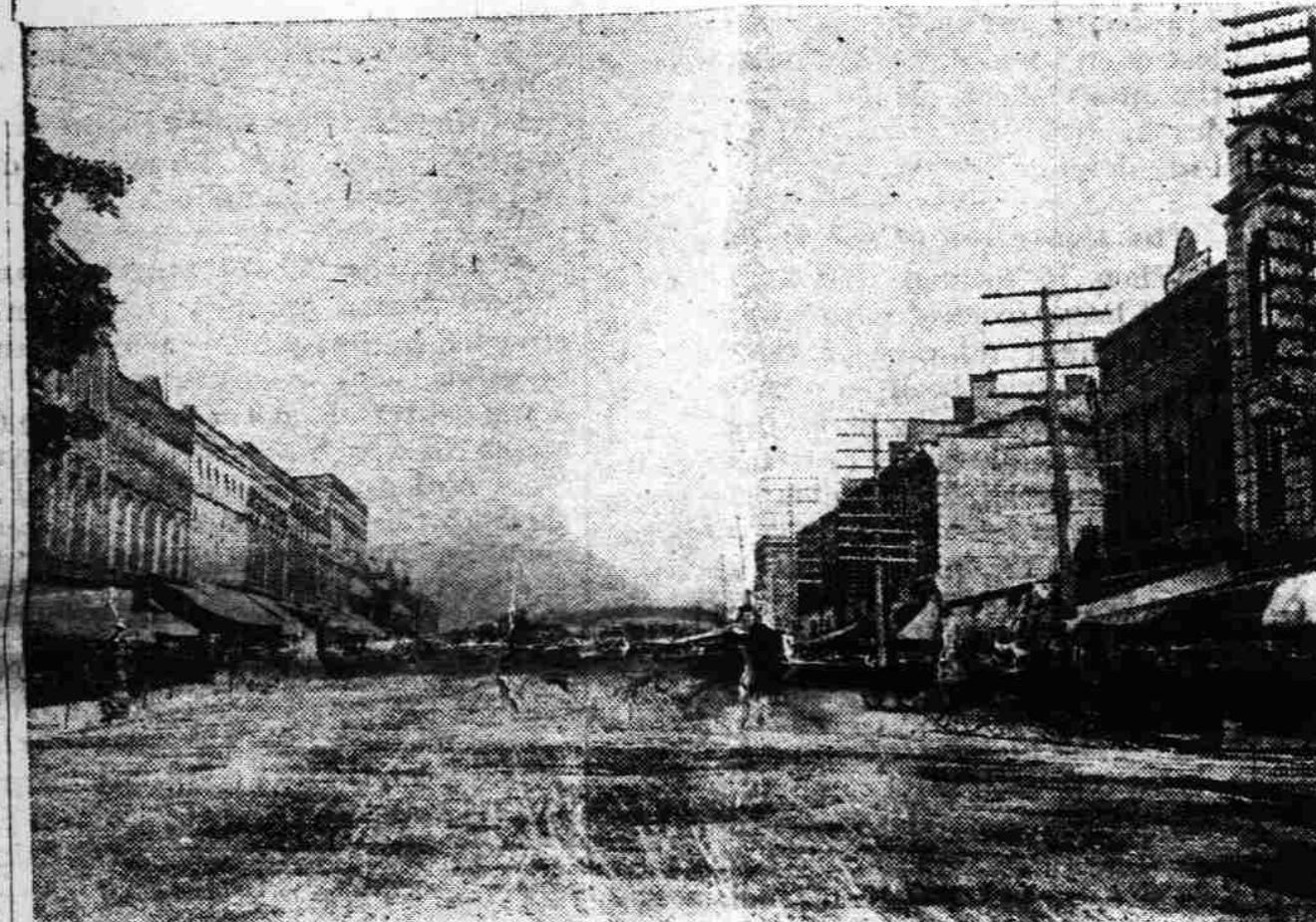
Main street looking North from Central Hotel, showing new buildings in course of erection.
