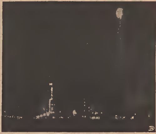
PORT ARTHUR, TEX.—A fitting symbol of fire prevention, this 200 ft. refinery flare burns up fire hazards before they start. Far from wasting gas—as often wrongly supposed—it actually is a safety valve. During emergencies it consumes excess gases before they can build up into explosive concentrations; stands 24-hour guard to burn off possibly dangerous fumes. This unusual view of night light at the Gulf Oil refinery here was taken in a 10-second exposure at F.11 with fast panchromatic film.
