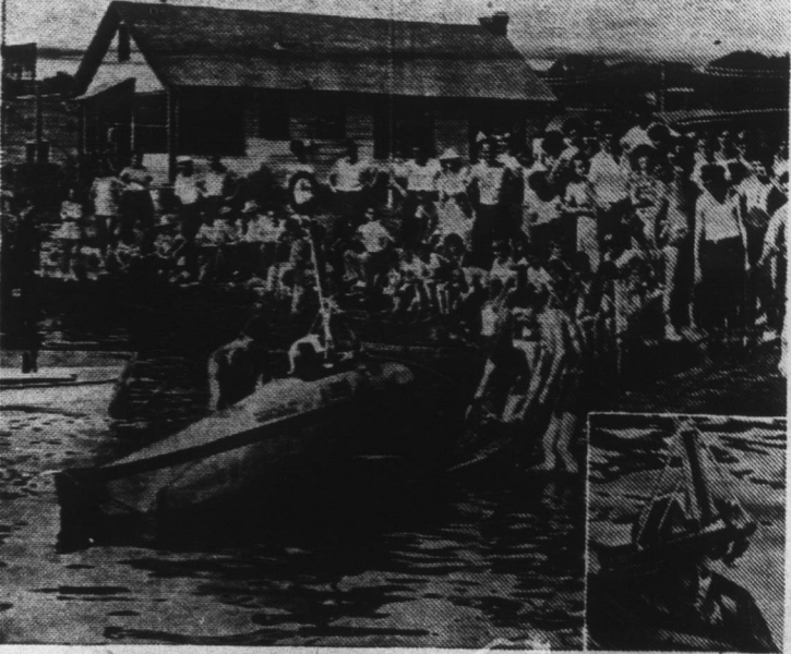
Barney Connett of Chicago, master and crew of an 11-foot subm., previous to making a successful test dive in the salt water of the Hudson river in Yonkers, N. Y. Connett, in his homemade sub, has made approximately 600 dives, once crossing Lake Michigan under water from Chicago to Michigan City, Ind., a distance of 37 miles. The sub is powered by two sets of batteries and has all the usual submarine equipment.
