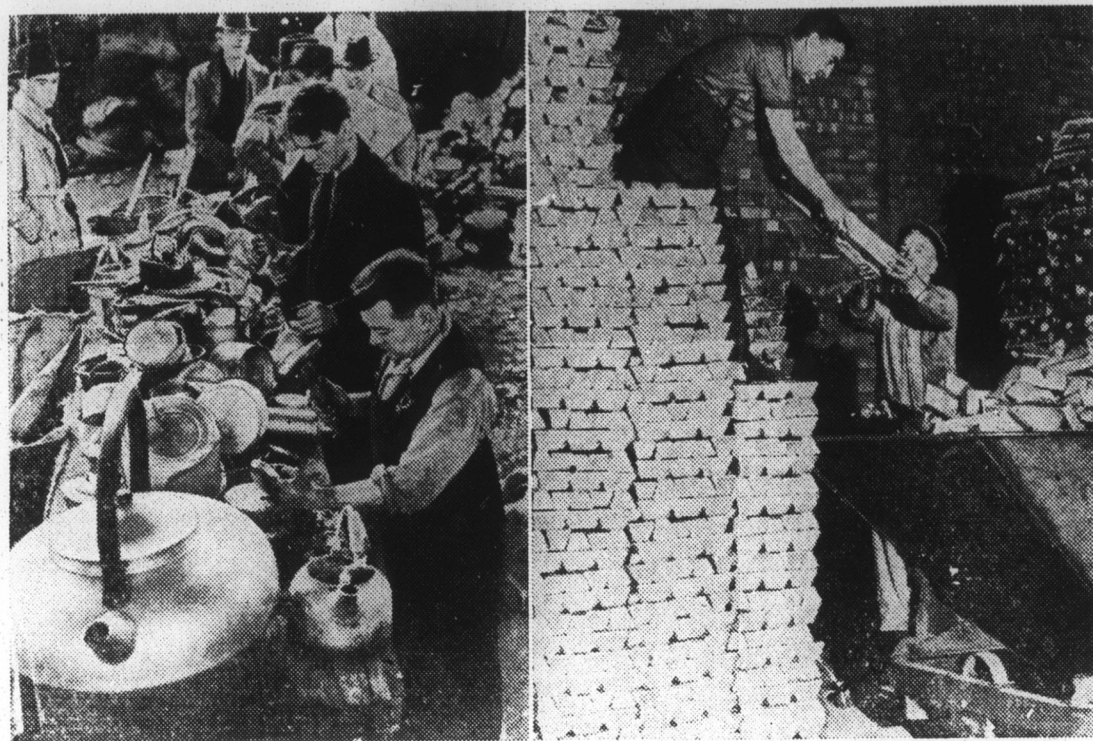
A government appeal for aluminum pots and pans brought thousands of tons of these kitchen utensils from all over England into the rapacious maw of Britain's war machine. From sitting on fires these pots and pans will go to cloud-hopping in defense of the tight little island. At left, workmen are cleaning the aluminum scrap. Right, tons of ingots, once stewpots, on their way to become "Spitfires" and Hurricane planes.
