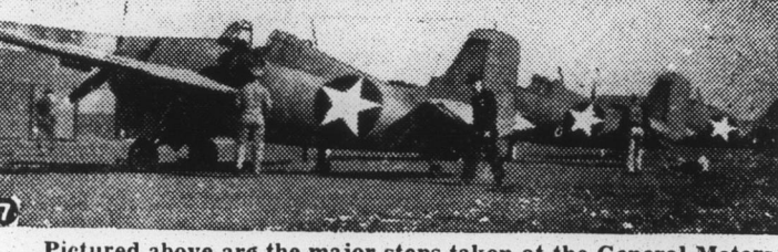
Pictured above are the major steps taken at the General Motors Eastern Aircraft plant at Linden, N. J., in the first complete conversion of an automotive plant to the production of finished airplanes. From top to bottom: 1—The old auto assembly line. 2—Demolition. 3—Stripped plant. 4—Planning. 5—Training. 6—The new airplane assembly line. 7—Flyway. In addition to the Linden factory, four other Eastern Aircraft plants of G. M. which were manufacturing automotive parts or assembling automobiles a year ago are now producing fighter planes and torpedo bombers for the U. S. Navy. It was necessary to rip out all the automotive equipment, redesign many sections of the five plants and engineer new processes to take advantage, where possible, of the mass production experience of automobile days.
