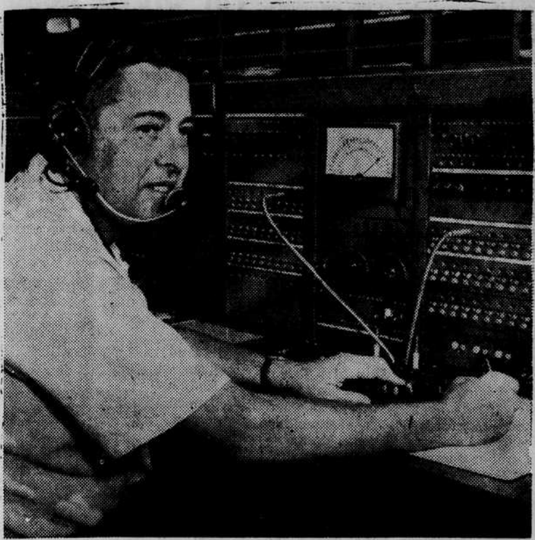
Guided by electronic "eyes and ears", the test deskman spots line troubles at once and gets repairmen there quickly, often before service is actually interrupted.
