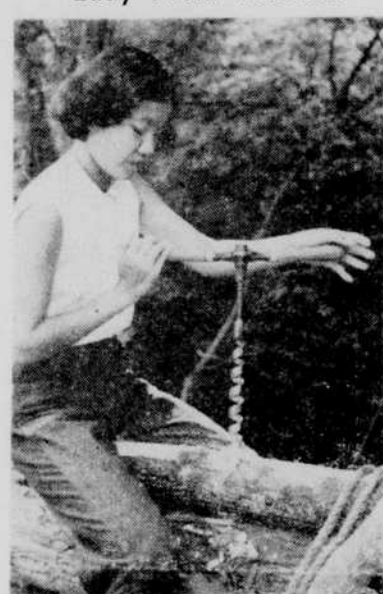
This young lady from Thailand is trying out a brace and bit as she prepares a log for one of the buildings at the Work Camp in Buckeye Cove. Leaders said that outstanding during the weeks the camp was in session was the spirit of willingness and cooperation which existed. This student from the Far East exhibits this as she acquires new skills.
