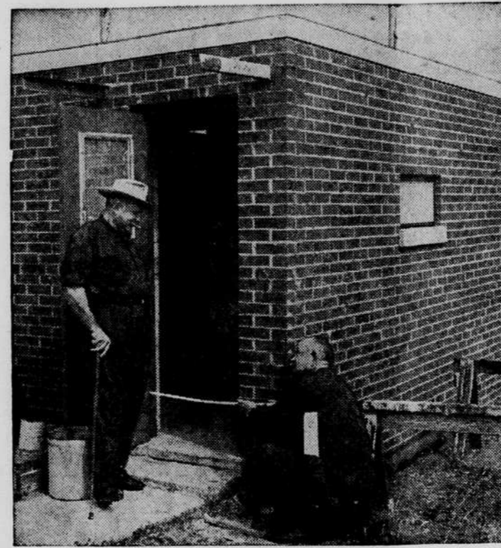
ENGINEERING ADVICE on how to add an entrance baffle to his new fallout shelter is obtained by Carl L. Underhill (left), of Raleigh, from Archie W. Green, Jr., engineer for the North Carolina Civil Defense agency. Underhill discovered that a baffle was needed to block dangerous levels of radiation which, after nuclear attack, could penetrate a normal door of this $1,000 shelter. Green was hired early in 1961 under a Federal program to pay half the costs of new civil defense employees. (OCDM Photo)
