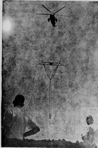
A new aluminum power transmission tower which can be flown intact into remote areas and lowered into place by belicopter is shown during eccent demonstration at Stratford, Conn. Known as the Alcan Design Y-Tower, it offers savings in construction of high-voltage transmission
